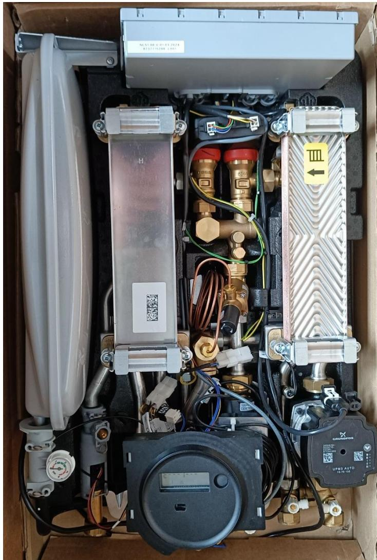
Figure 21 - HIU with outer case removed
