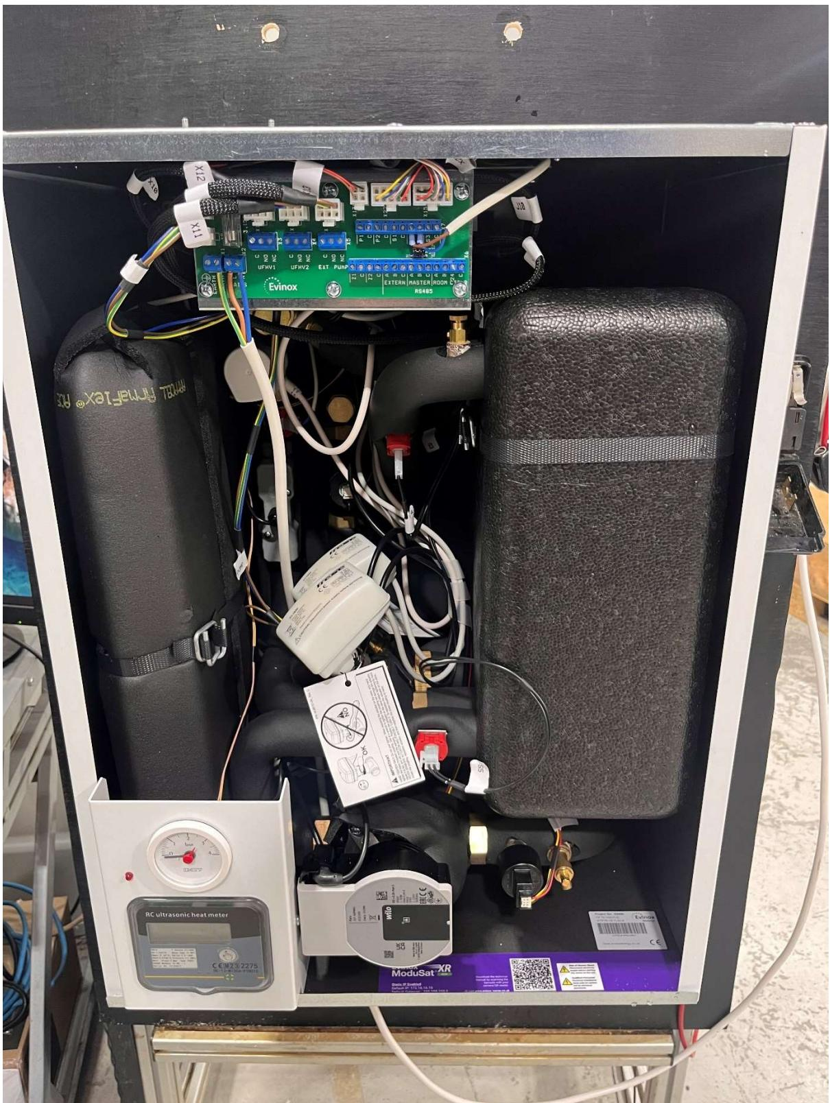
Figure 12 - HIU with outer case removed
