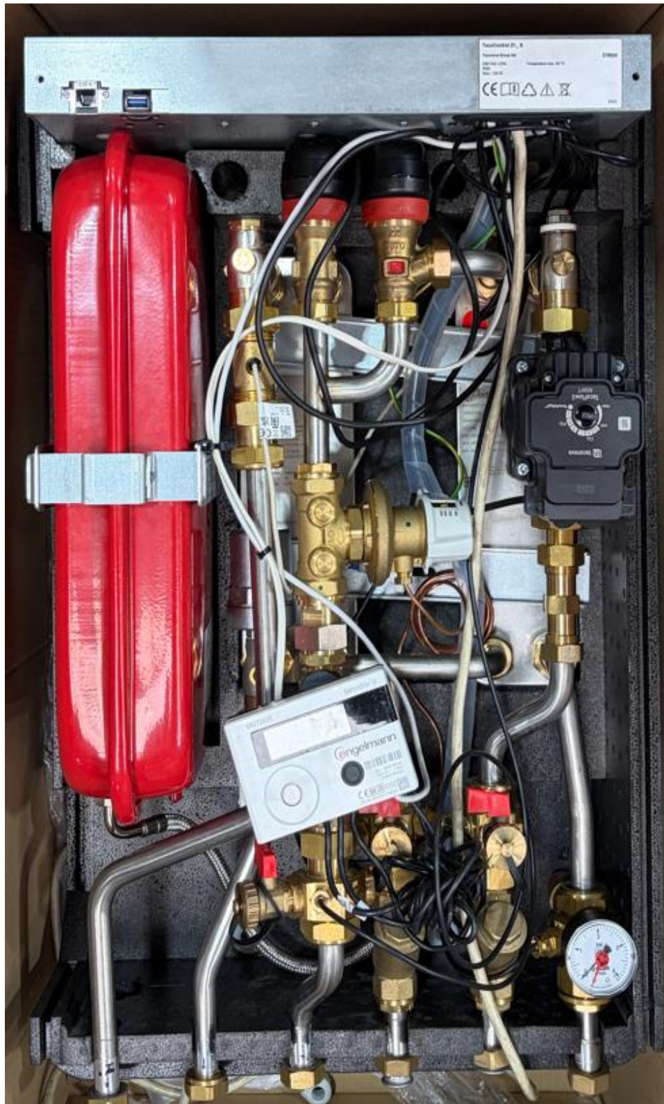
Figure 21 - HIU with Outer Case Removed
