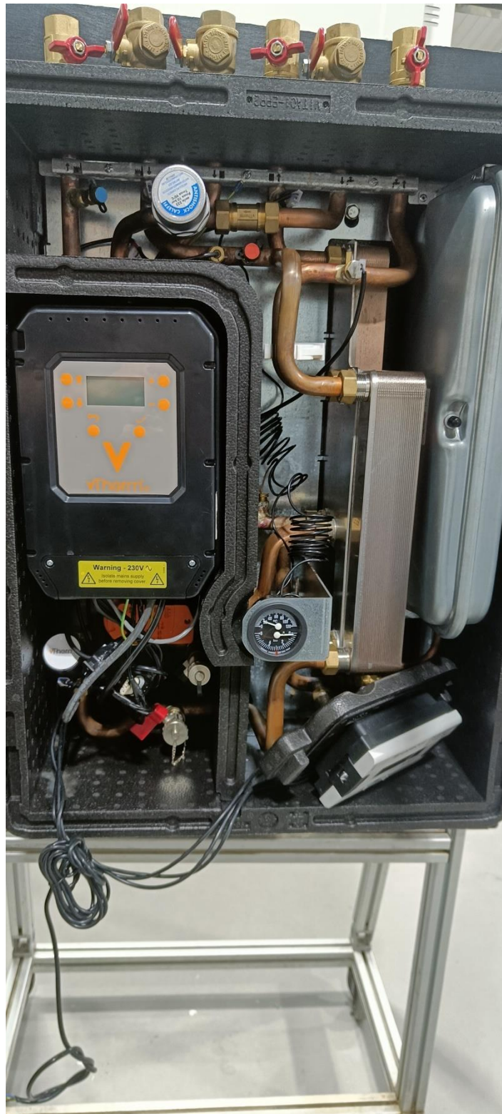
Figure 21 - HIU with Outer Case Removed
