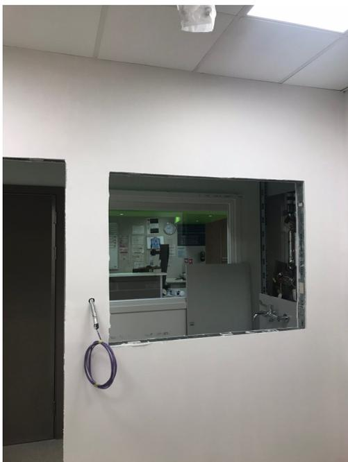
The dividing walls were built with standard construction materials together with hygiene cladding, with wash stations, Basins and taps installed in accordance with HTM Standards.
